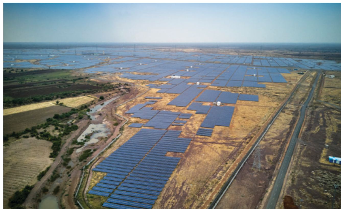
Sterling and Wilson Renewable Energy Limited commissioned 195 MW Solar Power Plant for Softbank in Kurnool, Andhra Pradesh
