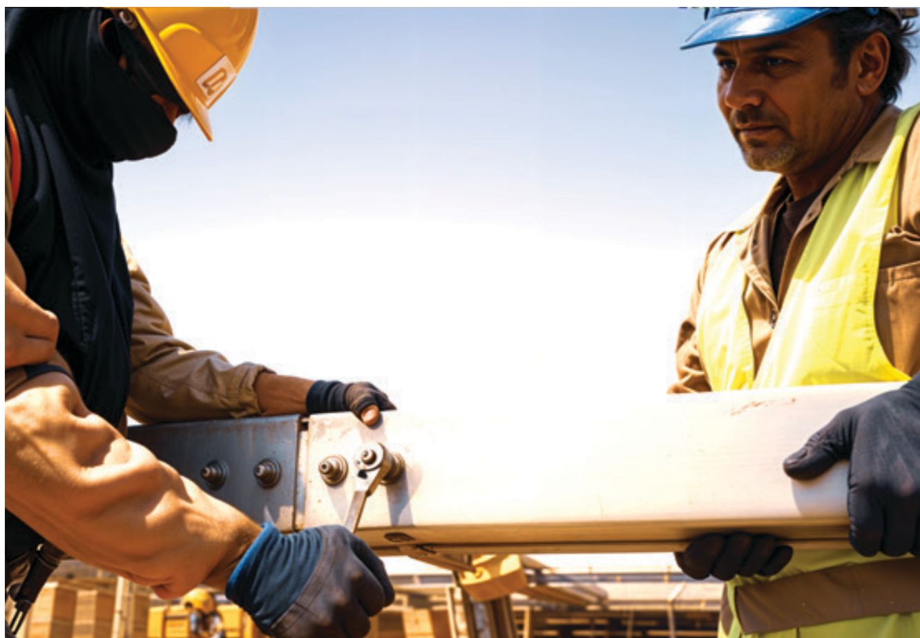
Workers at the Abu Dhabi, UAE project site
