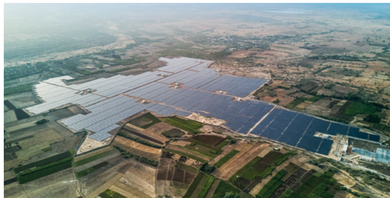
40 MW (AC) Hindupur Solar Park commissioned by Sterling and Wilson Renewable Energy Limited
